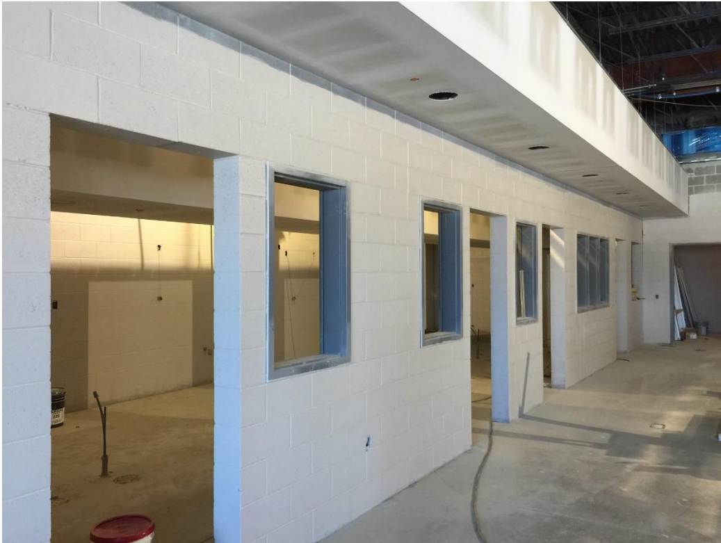
Multi-purpose room and kitchen painted
