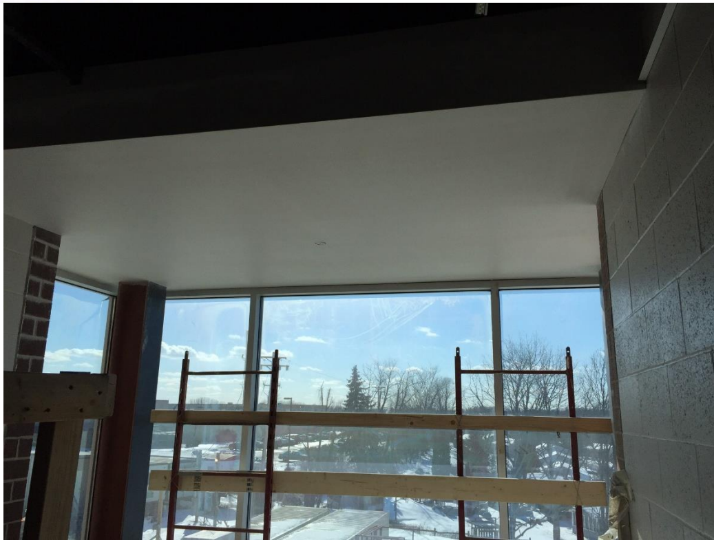
Bulk head in area B stairwell
