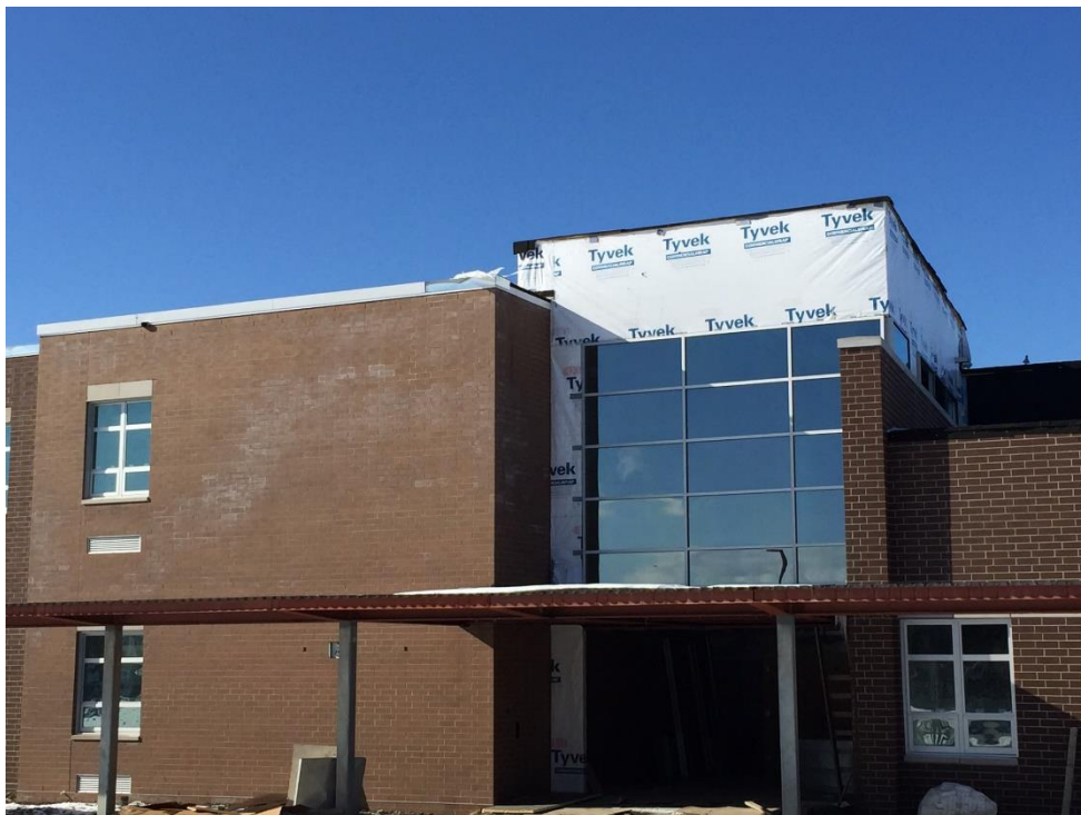
Store front glass and roof coping
